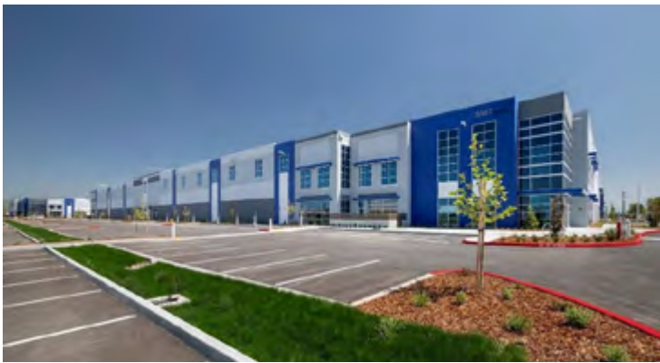
Cepheid leased 178,910 SF at 44509 Pacific Commons Boulevard, Fremont
