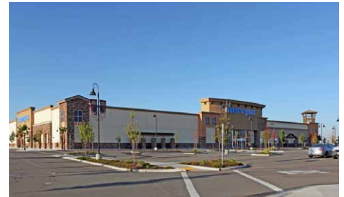
This former Mervyn's department store at Blue Oaks Town Center in Rocklin was recently leased to SR Entertainment Group. The 80,000 square foot building is being converted to a 16-screen theater. Our sources have told us that the conversion costs will likely exceed $8.5 million and that these costs are being split between the landlord and the tenant.
