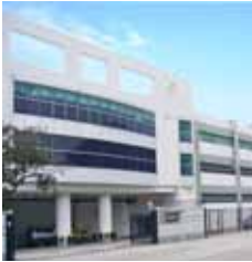
No. 2 Chun Yat Street, Tseung Kwan O Ind. Estate Sold 360,000 sq ft
