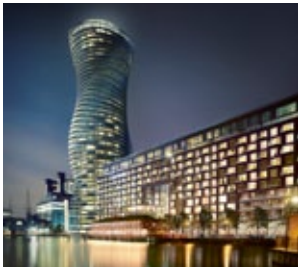
Baltimore Wharf, London, UK
