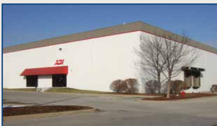
Honeywell International Owned by Dixie Real Properties, LLC
