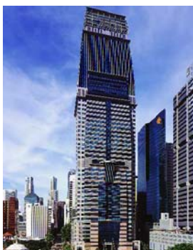
Capital Tower in Singapore is a benchmark for Intelligent Buildings in Asia.
