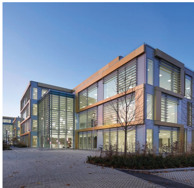
Bourne Business Park, Weybridge
