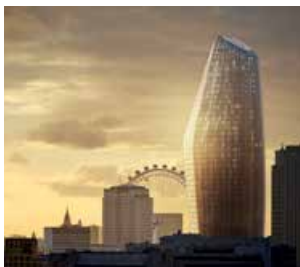
One Blackfriars, London, UK
